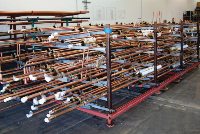
Figure 4. Prefabricated piping sections.
